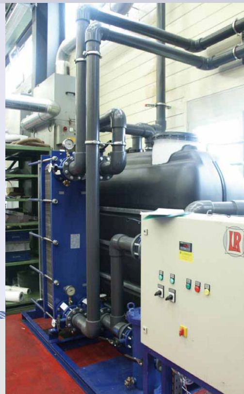
Cooling of lubricating oil for extruding presses.
